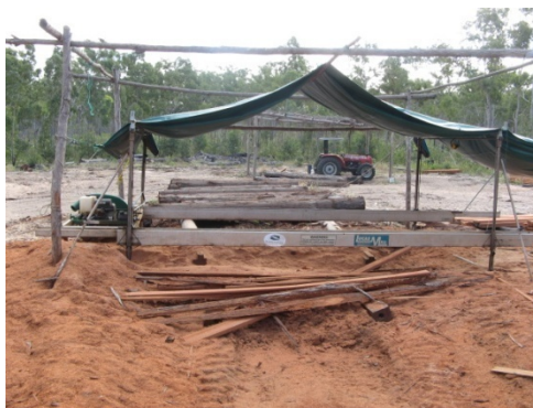
FIG. 1: TIMBER MILLING NEAR GARRATHIYA
